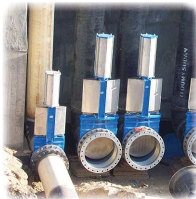
Mixing chamber installation
